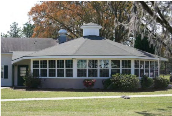
(They will begin the new roof this week)
